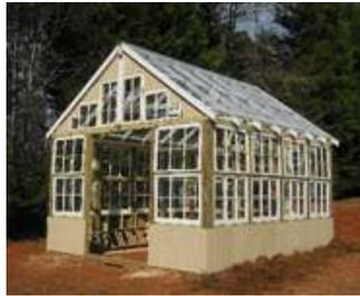
Typically, the windows themselves will not hold the weight of the roof so some type of framing structure will have to be incorporated into the design.
